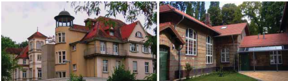
Figure 2 Dedicated Bernstein Center buildings in Freiburg (left) and Berlin (right).
